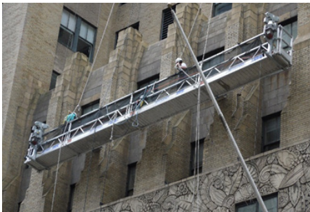
Walk-thru 'C' stirrup on swing stage scaffolding
