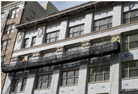
Cross beam swing stage scaffolding
