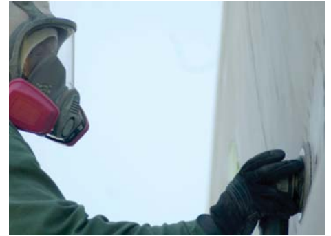
Figure 24. Dust from sanding
