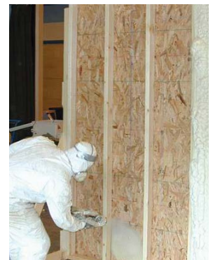
Figure 36. JobCorp student using a soy-based spray foam.
