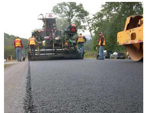
Figure 25. Vapors and dust from asphalt
