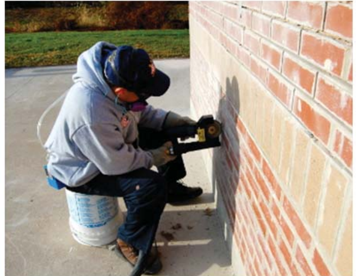
Figure 40. Tuck-pointing with controls
