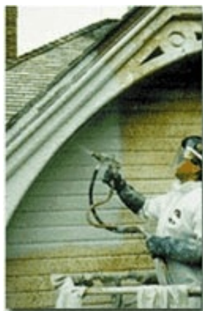
Applying Peel Away ST-1
