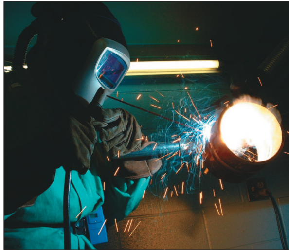
Fred Weber, a union instructor, TIG-welds pipe during the evaluation of a portable local-exhaust ventilation unit.
