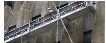
Walk-thru 'C' stirrup on swing stage scaffolding
