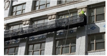
Cross beam swing stage scaffolding
