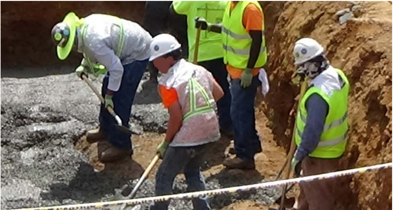
Figure 1. Poured-concrete foundation workers wearing the Aluminet and conventional vests during work.
